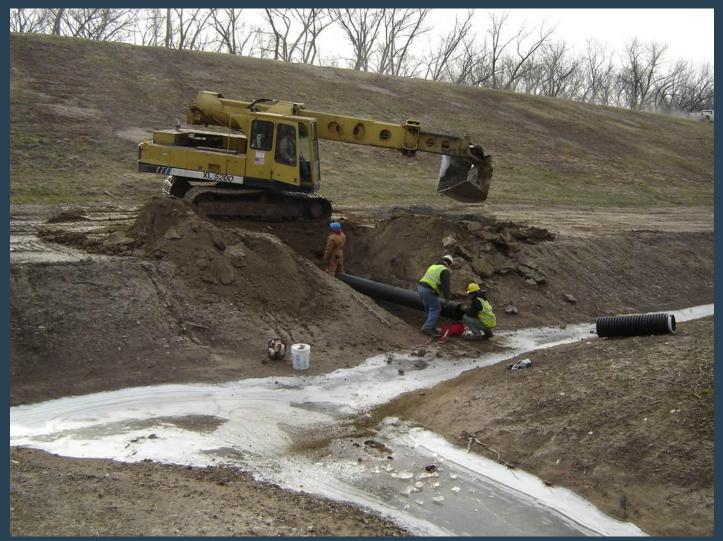
Lateral drain being repaired with HDPE sleeve
