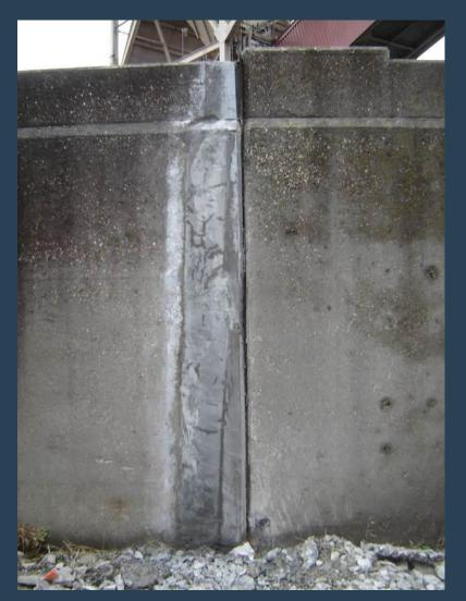
Repaired floodwall keyway near MIRA Powerplant
