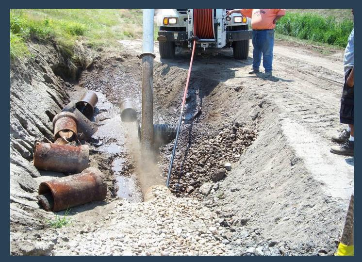
Toe drain clogged with sediment being cleaned
