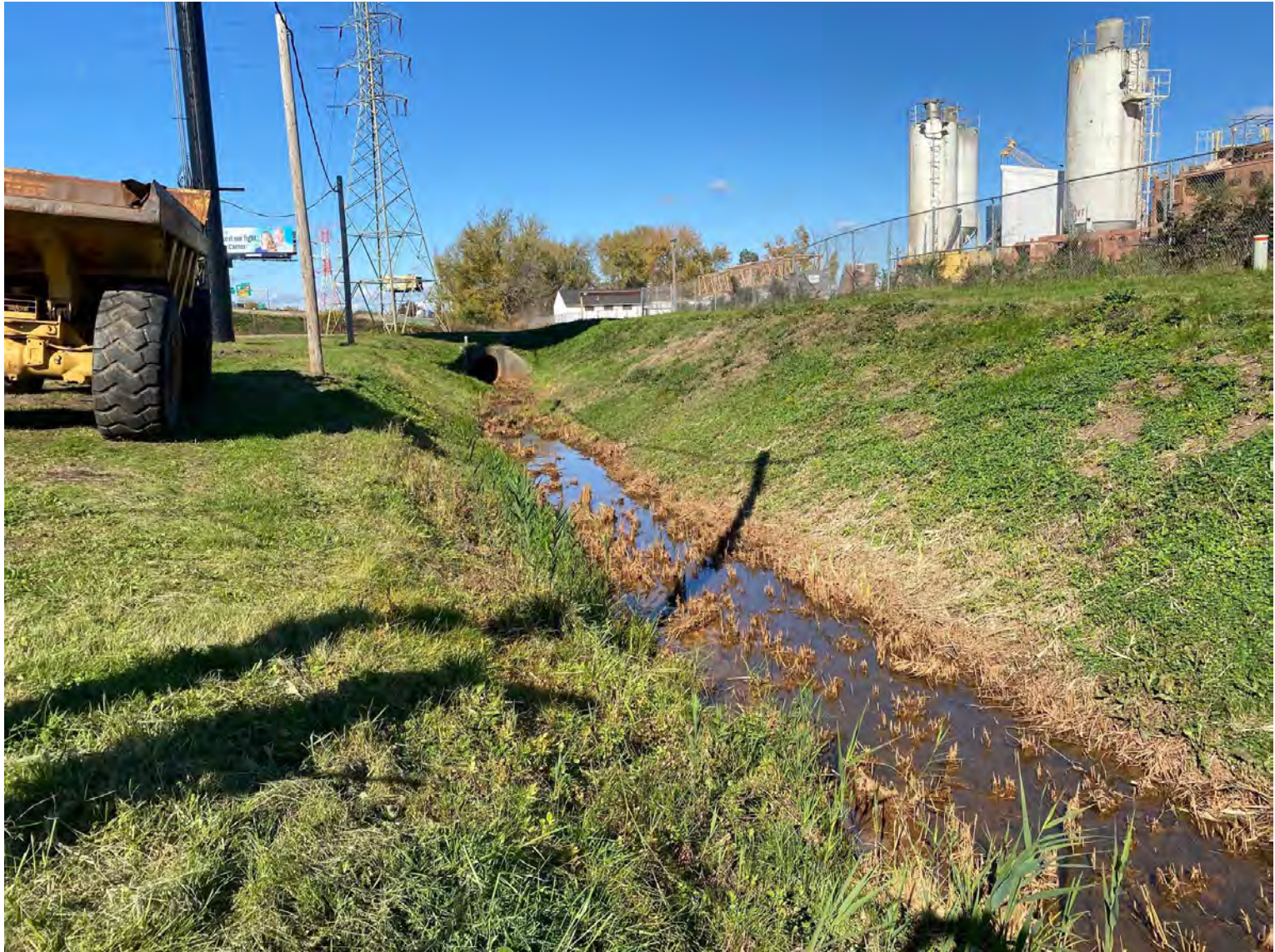
WETLAND FLAG SERIES 3 AREA LOCATED ADJACENT TO THE EAST OF I-91 LOOKING WEST.
