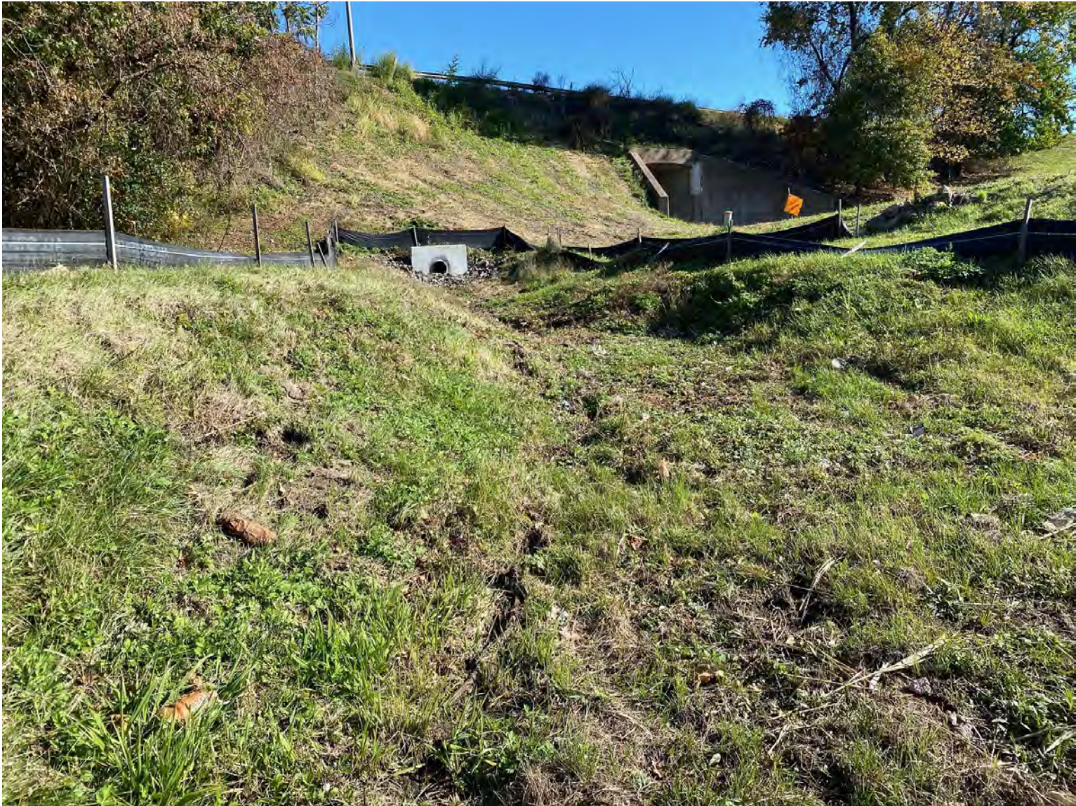
WETLAND FLAG SERIES 2 AREA LOCATED ADJACENT TO THE WEST OF I-91 AND EAST OF SERIES 1 WETLAND. VIEW LOOKING EAST TOWARD I-95.
