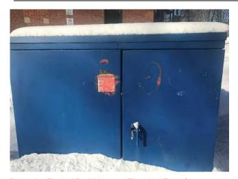
Photo 25: Typical Pad-Mounted Electrical Transformer.
