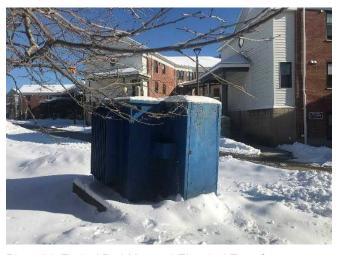
Photo 26: Typical Pad-Mounted Electrical Transformer.
