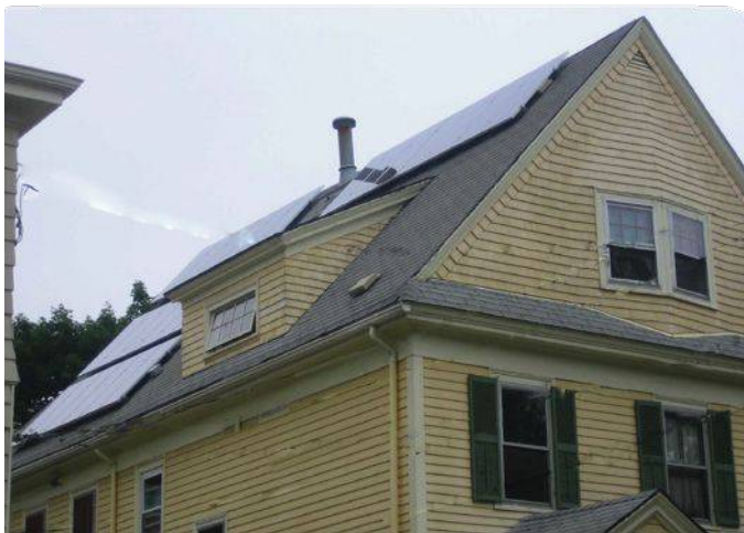
Figure D. Photovoltaic System on a Pitched Roof. The low profile and location of these solar panels make them unobtrusive, even though they are visible from the public right of way. (Photo courtesy National Alliance of Preservation Commissions.)
