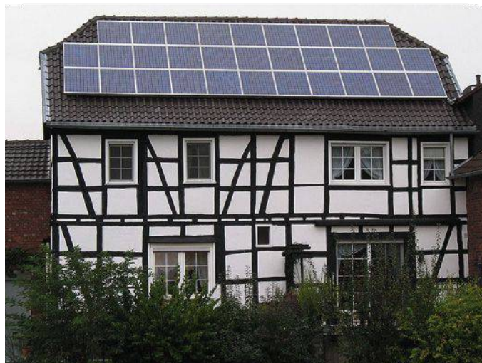
Figure A. Building-Mounted Solar. (Photo courtesy National Alliance of Preservation Commissions.)
